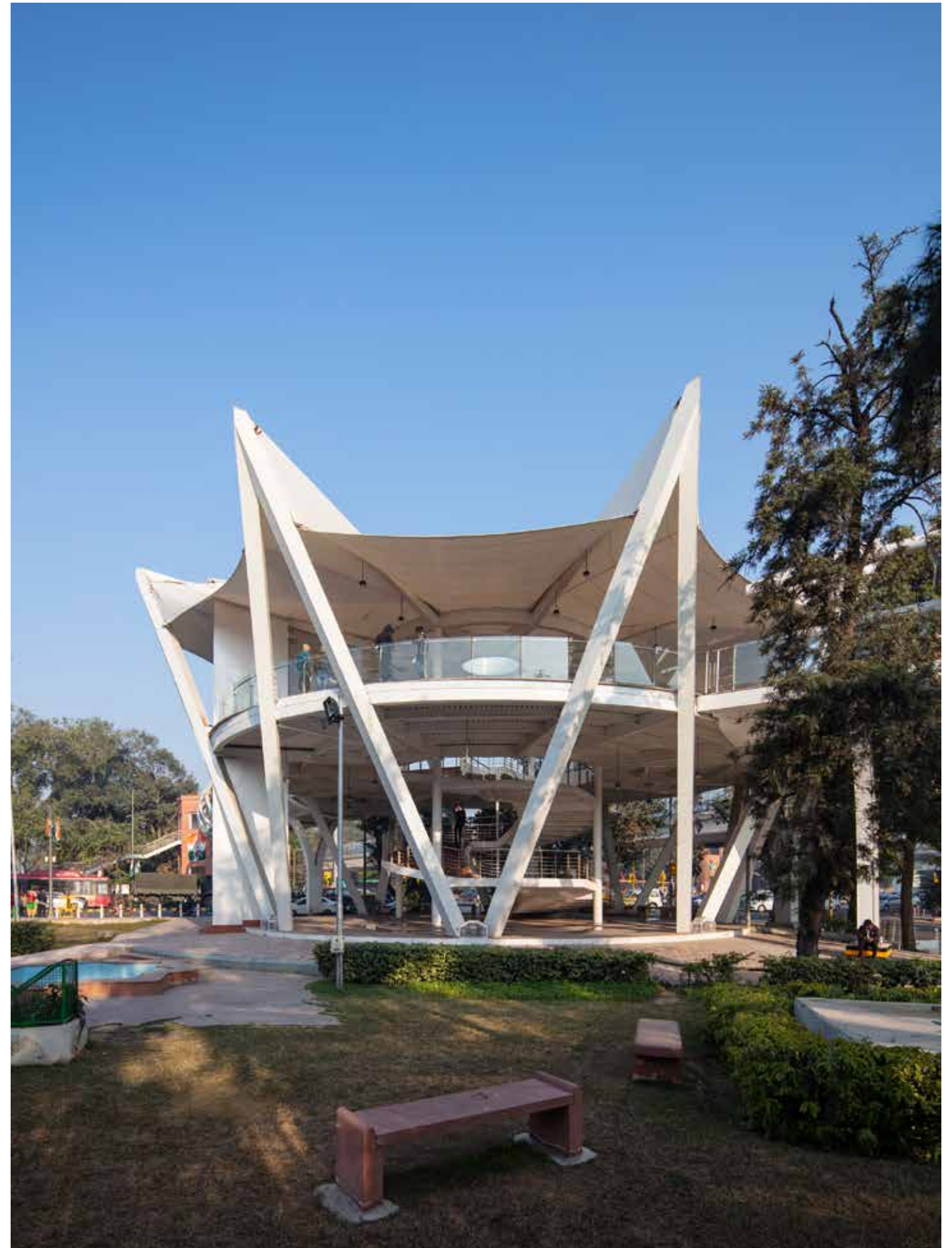
The octagonal unit consists of steel crowns and uses granite flooring and S.S. glass in the railing.
