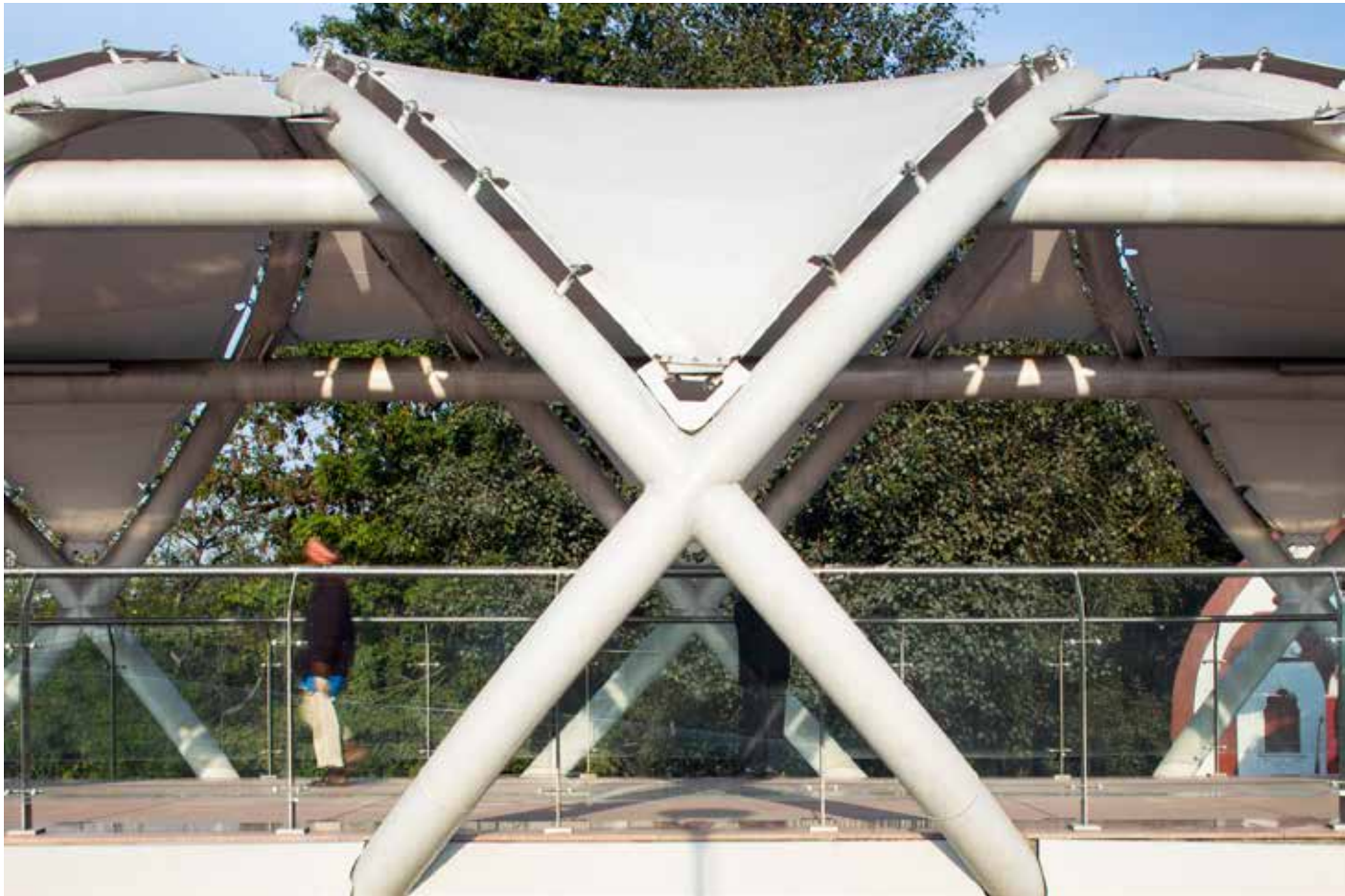
52 The criss-cross boot lace trusses are covered with tensile fabrics, resulting in the unique silhouette of the skywalk.
